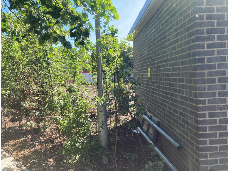
Fig 4: Front of sub-station with new planting in front
