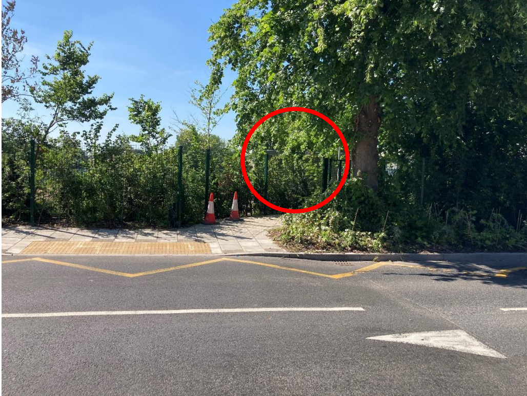
Fig 5: View from Chislehurst Road with location of sub-station circled in red
